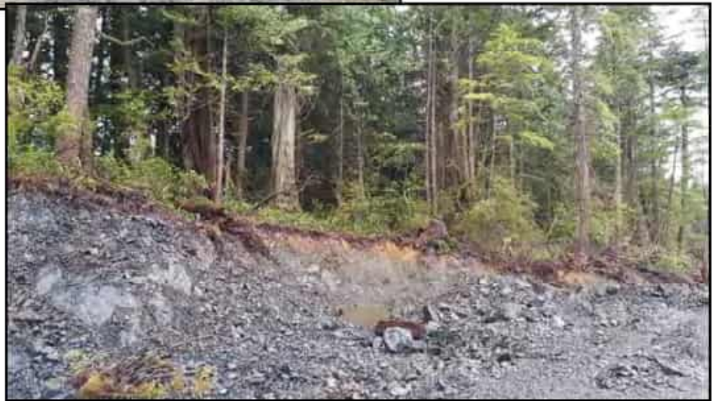
Photo 6: View along main access road; south end of development. Road cleared to edge of 30m highway setback.
