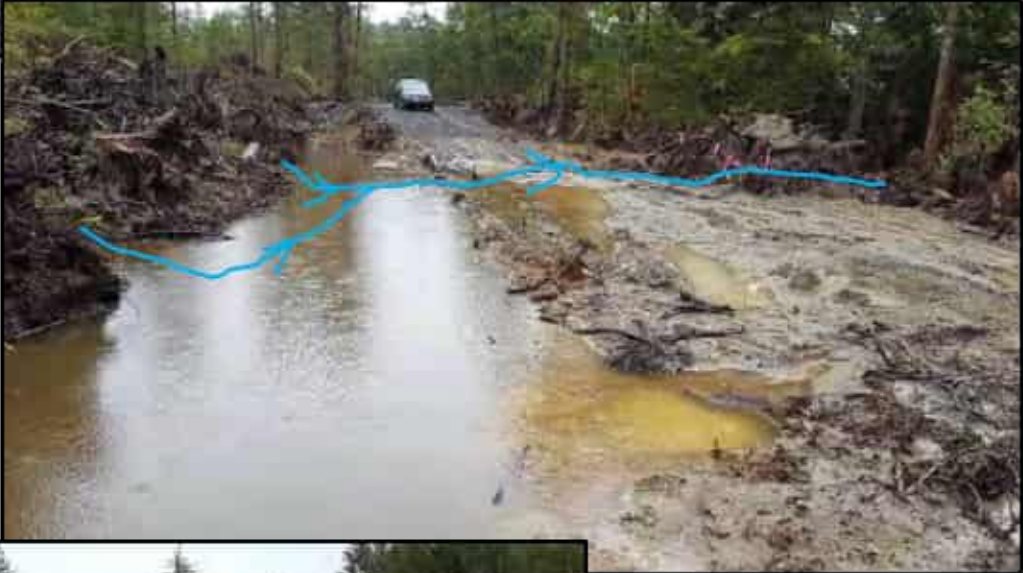
Photo 8: Impacted drainage. Area to be integrated into stormwater management plan for site. Overflow from the Middle Stream in the southern half of property.
