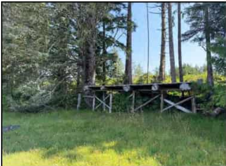
Photo 25. Narrow band of riparian trees along the northern tip of property. The wooden deck at shoreline built by previous owner without permit and should be removed.
