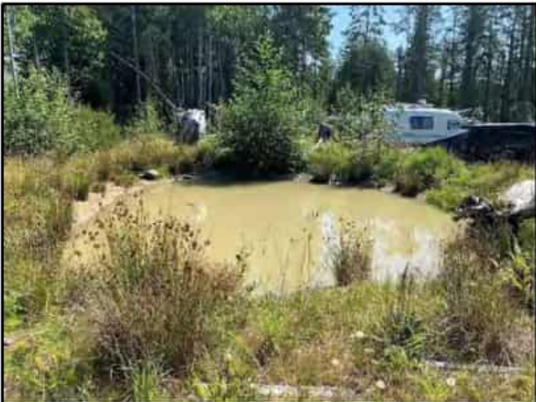
Photo 28. An excavated stormwater detention pond just south of the northern tip of the property in 30m setback to be infilled and revegetated.
