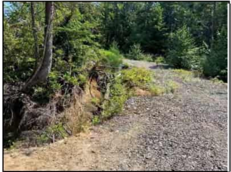
Photo 15. Gravel loop road through southern section of the site with deep ditches along the sides of the road.
